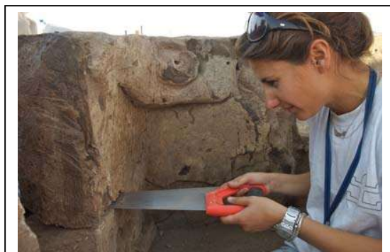
Figure 170: Cutting the plastered wall
